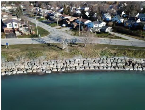
Municipal Shore Protection, Monk Street, Cobourg
