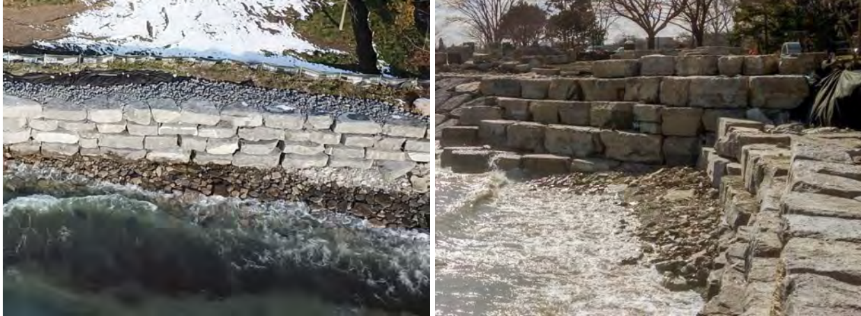
Figure 7.3 Sample armour stone seawalls on Lake Ontario
