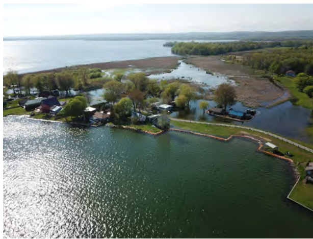
Flood Prone Properties, Evergreen Lane (May 2019)
