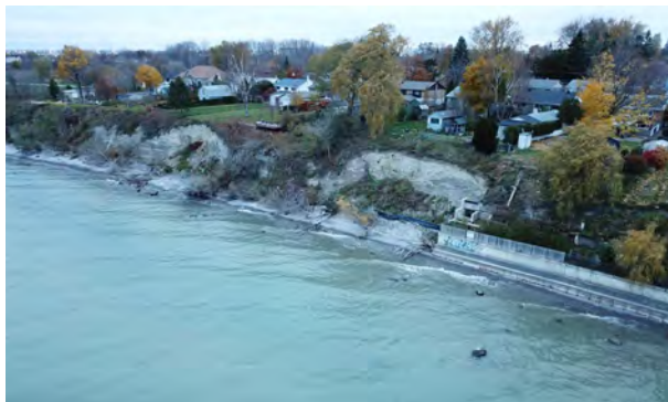
Eroding Bluff at Stone Street, Oshawa
