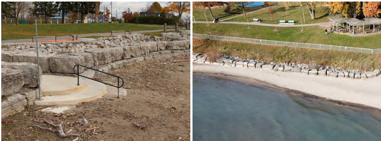
Figure 7.4 Sample armour stone beach curbs on Lake Ontario
